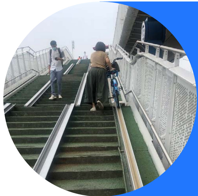
Beijing’s bicycle expressway is elevated above the street and features stairs with wheel ramps at entry points. Source: ITDP China
