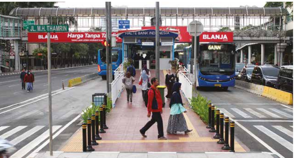
Important to Transjakarta's success has been creating and maintaining the proper BRT infrastructure, like off board ticketing and a dedicated lane.
